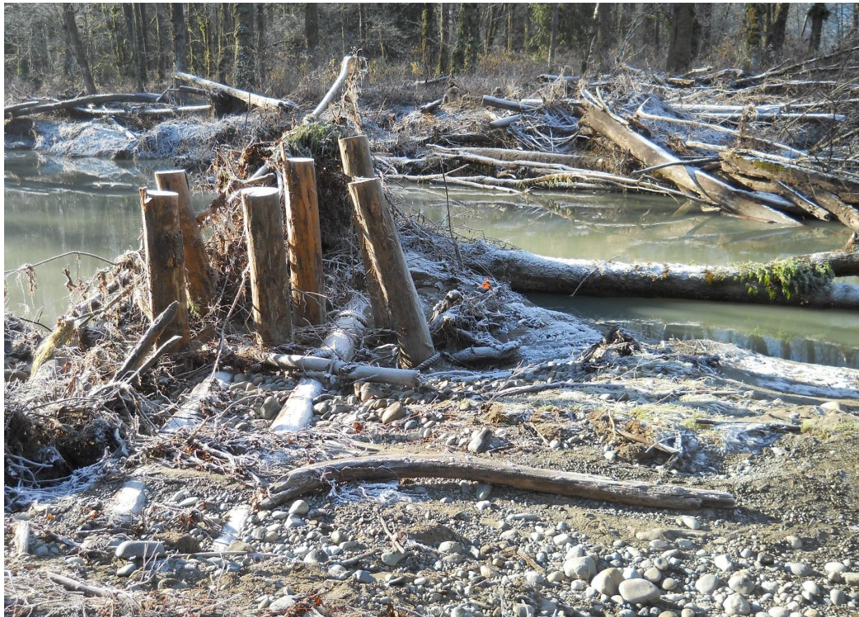
Figure 8. Example of small modular ELJ proposed for Illabot Creek, two years after construction.
